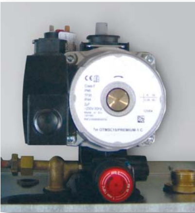
Pump body with built-in air vent
